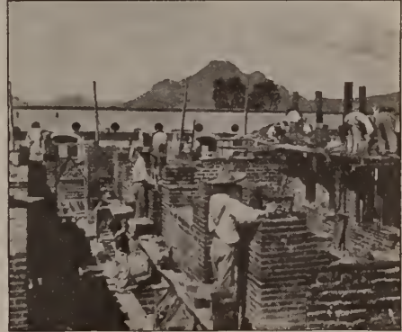
BUILDING THE NEW DORMITORY
